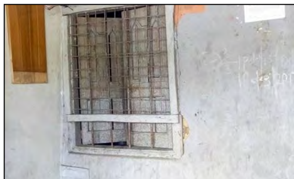
Figure 2: former PO window and post box
