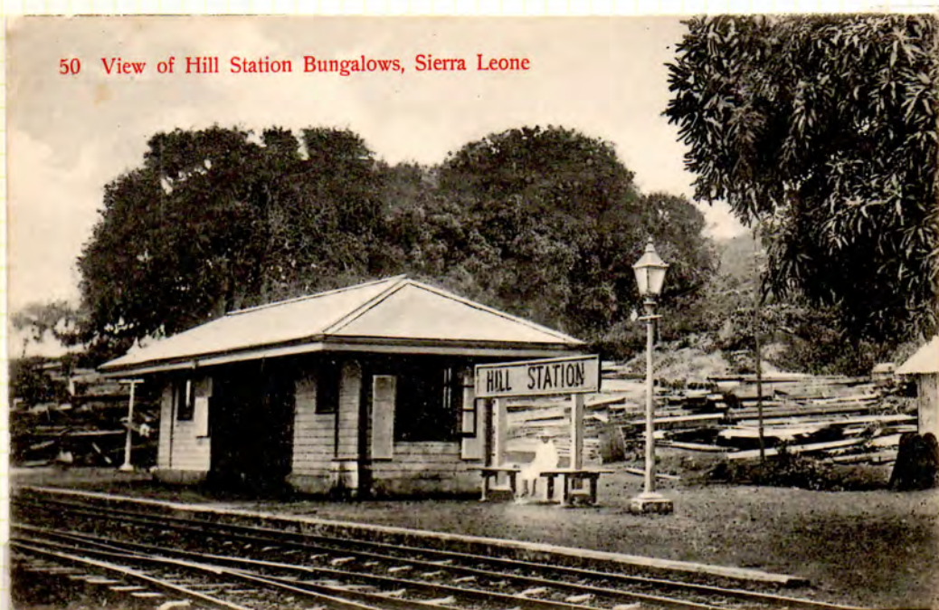
Hill Station. This was at the end of the Sierra Leone Mountain Railway
