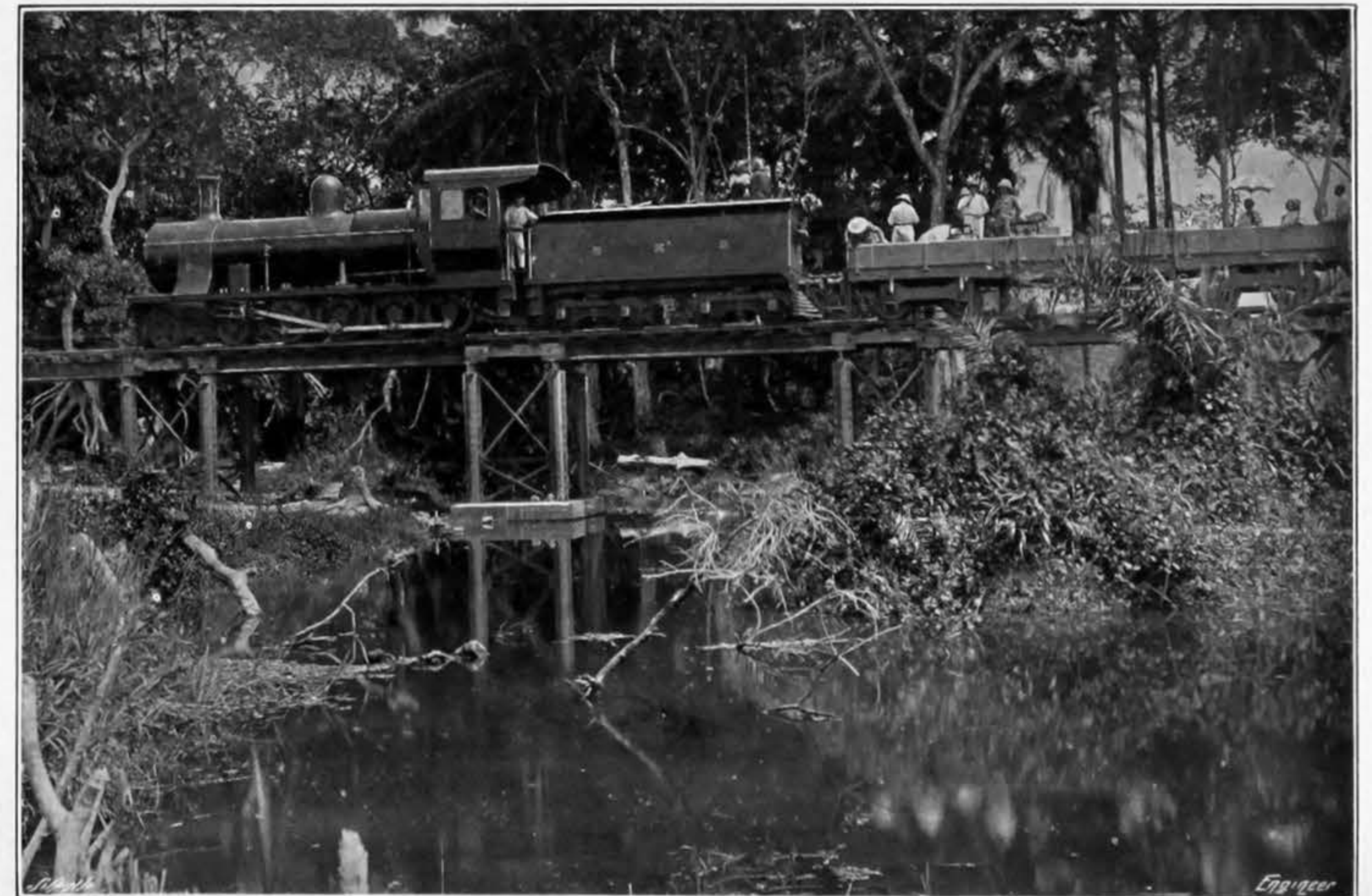
ENGINE OF THE EMIR CLASS ON STEEL BRIDGE
