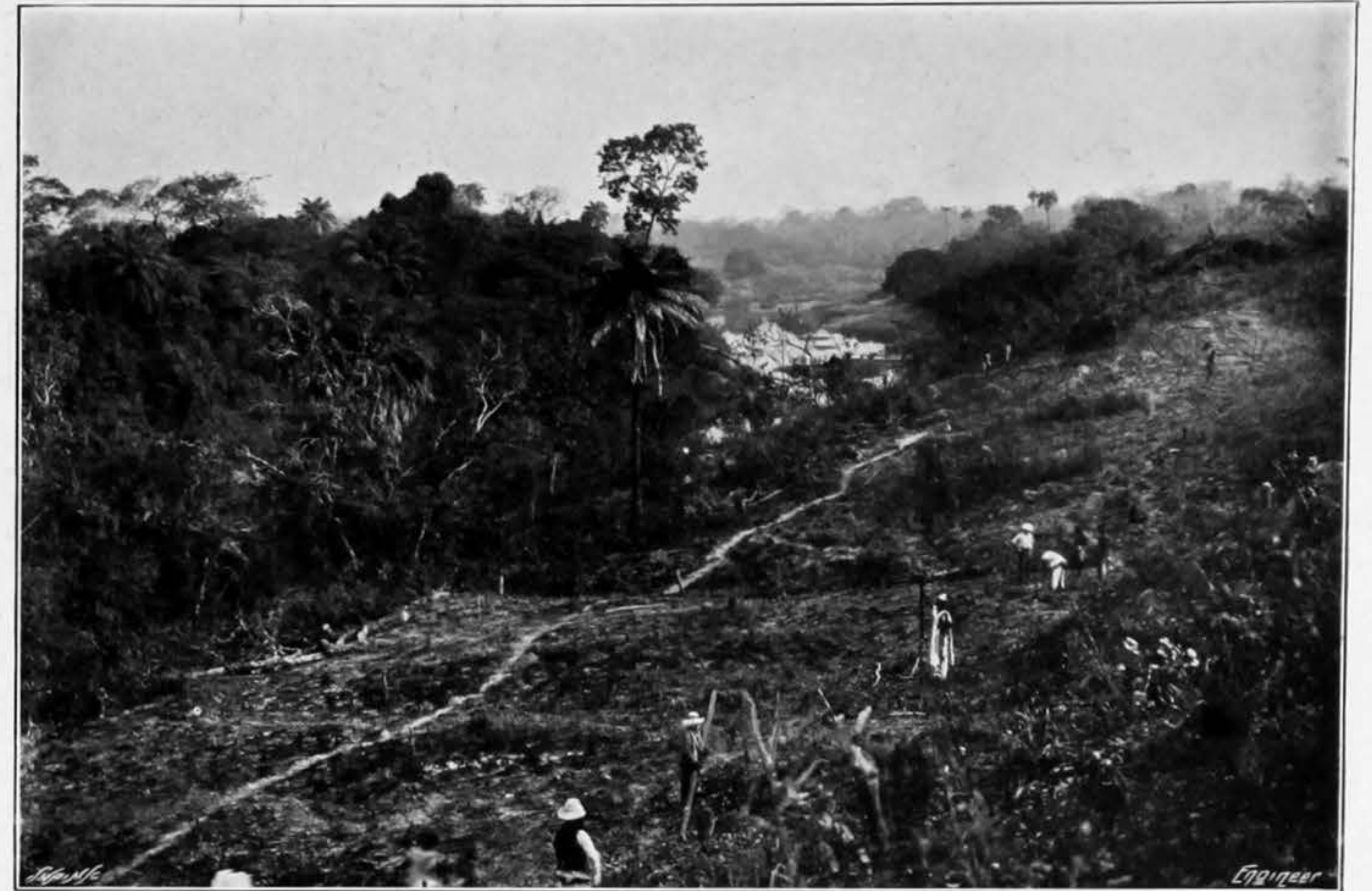
SETTING OUT EARTHWORK AT PATATIFI
