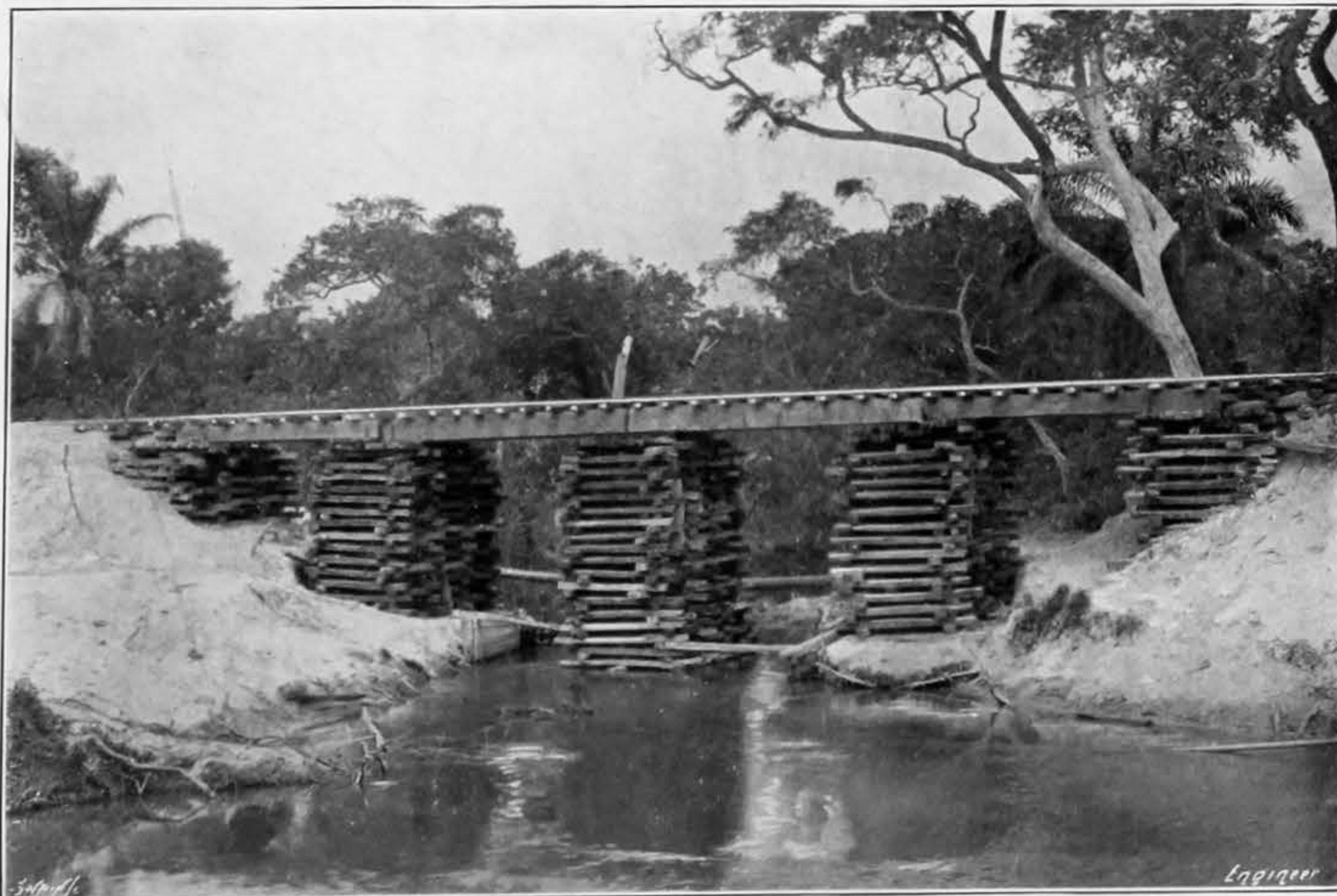
TEMPORARY BRIDGE OVER THE BAKOGI RIVER
