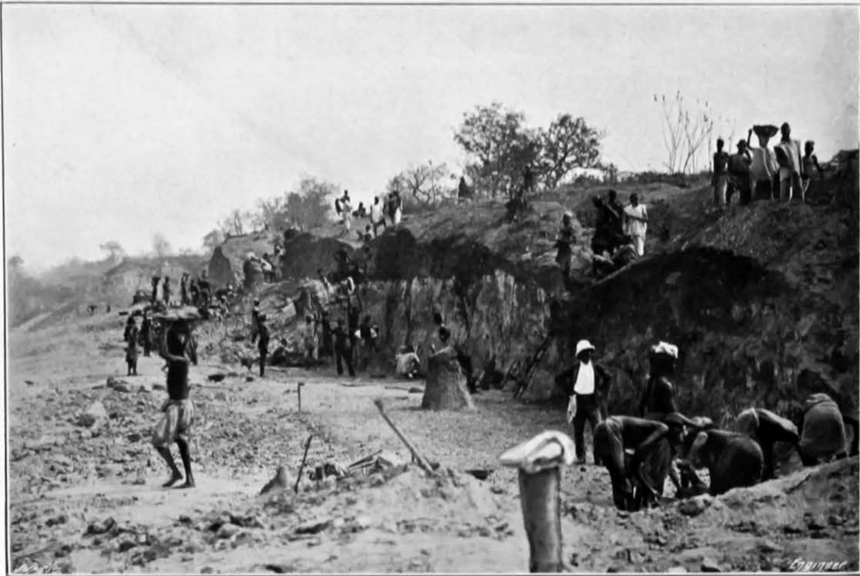
EARTHWORK IN PROGRESS AT PATATIFI BLUFF
